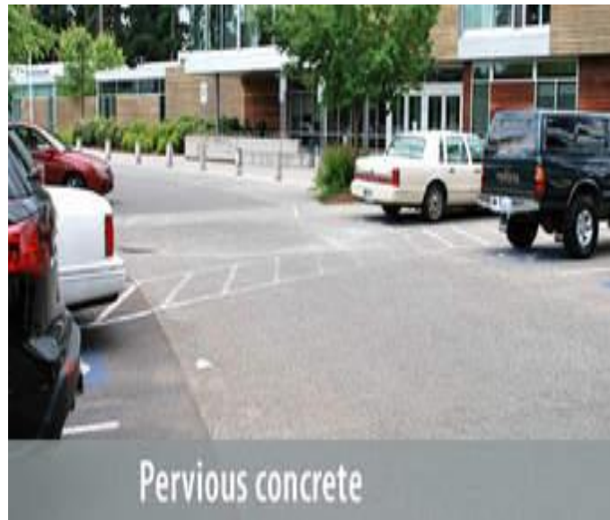
Fig.4 concrete laid on parking
