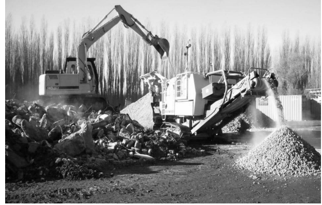
Fig. 4: C & D Wastes Converting to Aggregates
